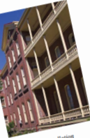
Figure 1: The installation of an exterior automatic fire sprinkler system for the historic multi-story porch allowed these important character-defining features to be retained to meet life and fire-safety code requirements. Photo: Robert Holcomb
